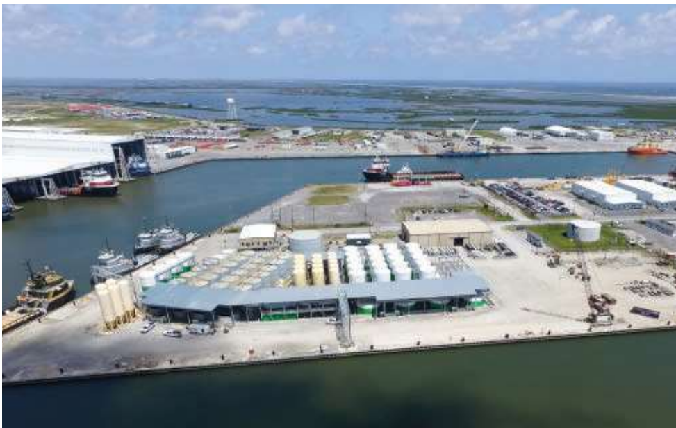
Newpark's completion-fluids facility in Port Fourchon incorporates the latest automated workflows and HSE standards.
