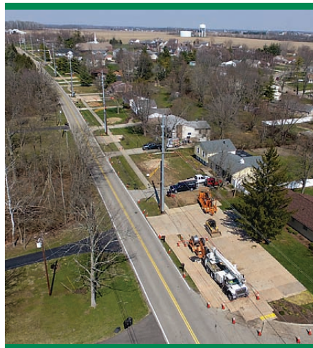
Access Road to Transmission Line Project
