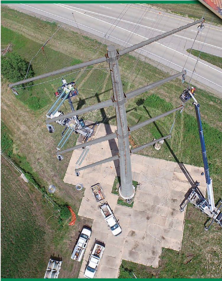
Stable Platform for Utility Projects
