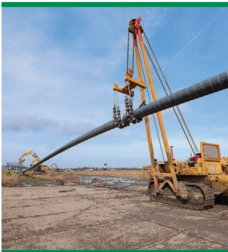
Pipeline Construction Project
