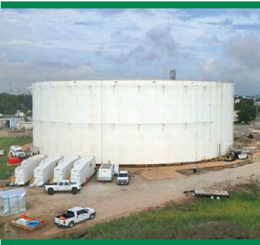
Tank Farm Project
