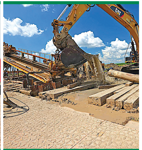
Directional Drilling Under Mississippi River
