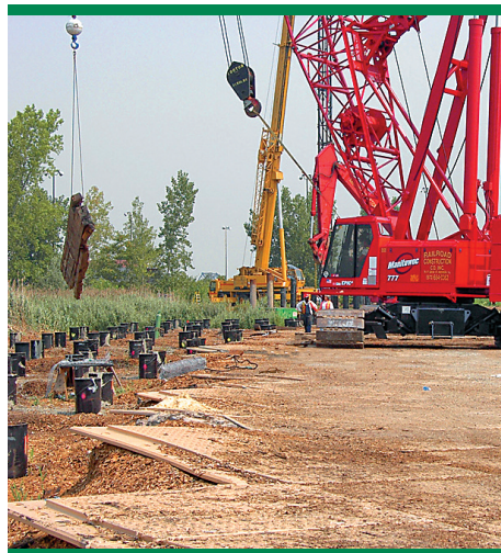
Pile Driving Project
