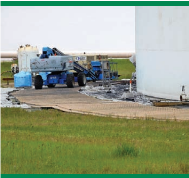
Maintenance Project in Louisiana
